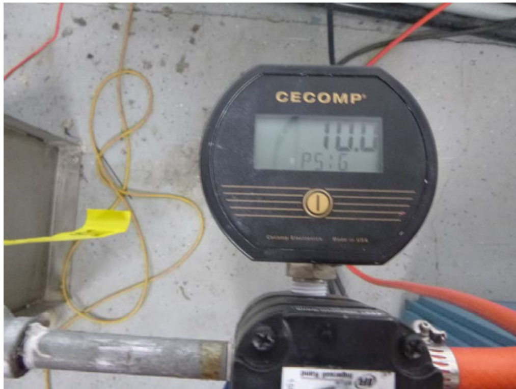
Overpressure Test Measurement
